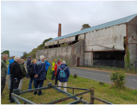
Glenarm Harbour Quarry workings
